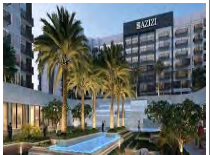
BEACH OASIS Residential Building (2B+G+09F) on Plot#6 by AZIZI, DU BAI
