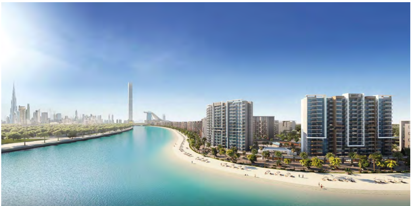
AZIZI Beachfront 01 - 2B + G + 20 - 3 TOWERS Residential Building, Dubai
