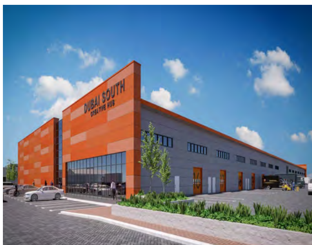
MULTIUSER WAREHOUSE DUBAI
